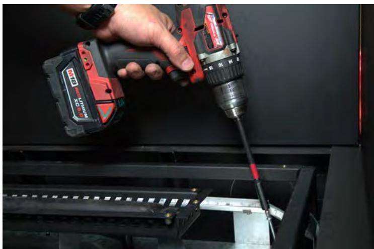
9. Locate the outlet in the back left corner of the fireplace. Using the appropriate knockout, bring your power into the fireplace. Make sure to secure your incoming power cord with the provided conduit clamps and connect the wire to the outlet using proper electrical connections and fittings (as shown next).
